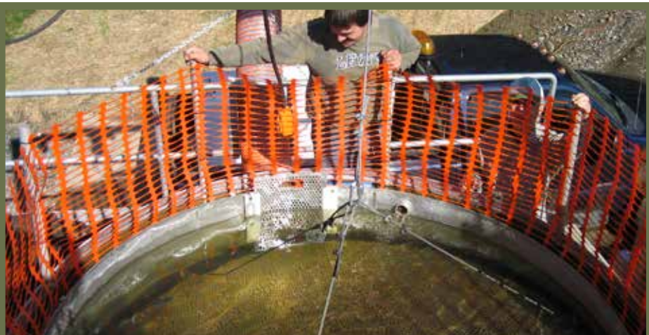
Clyde River fish ladder at the Clyde Pond Dam allows adult salmon to swim up the ladder and into a large holding tank. The salmon are then transported and released above the dam.
